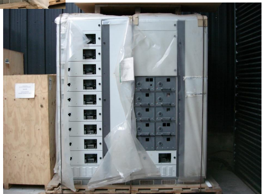
Pillars F8 & F9 (R8 & R9 at rear)
